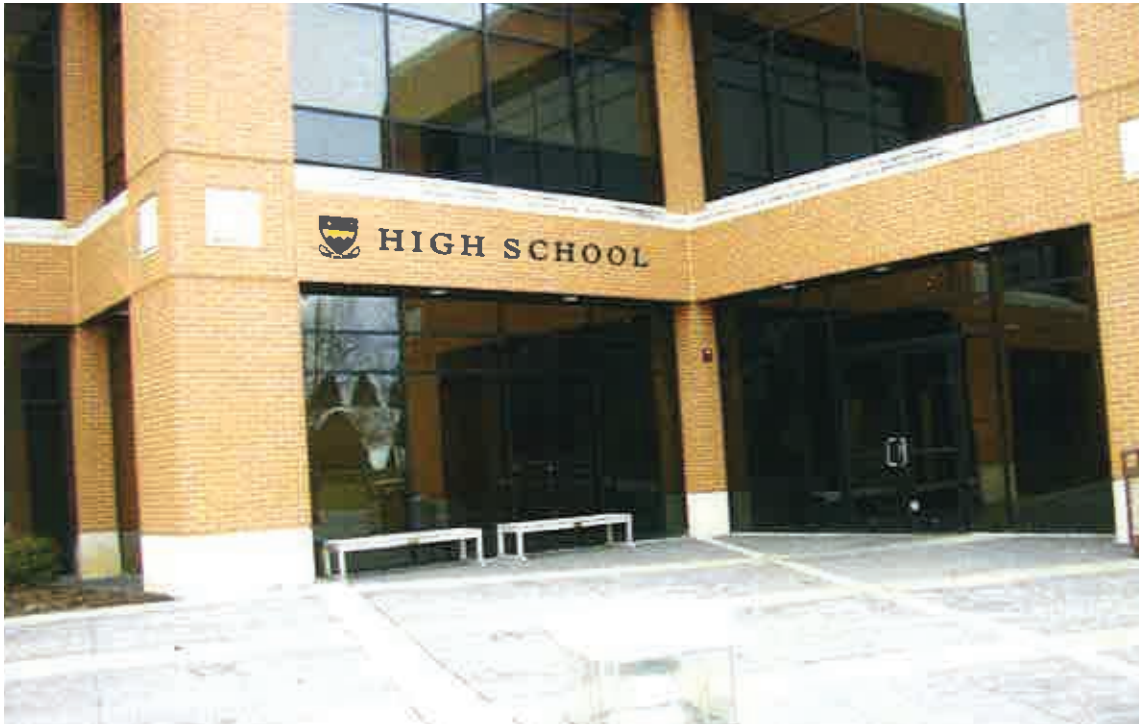
4 ENTRANCE @ HIGH SCHOOL
