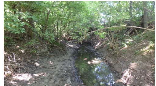
Figure ES-7: Bridge Downstream
