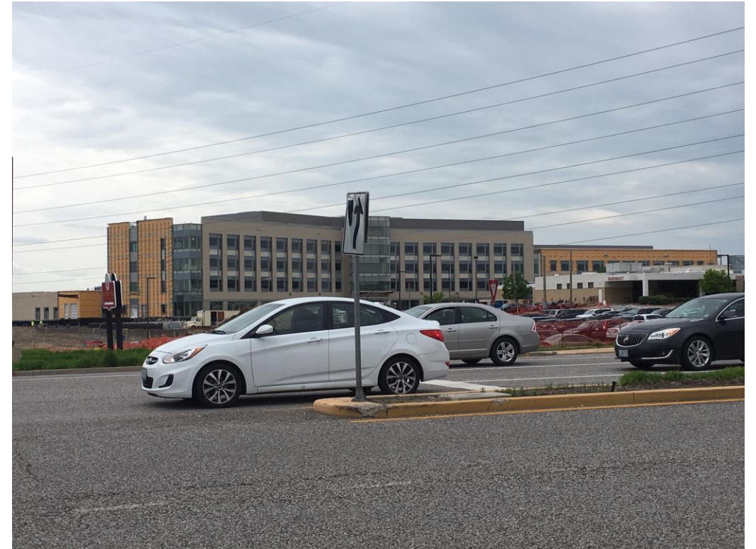
Barnes Jewish West County Hospital and Medical Office Building (Under Construction)
