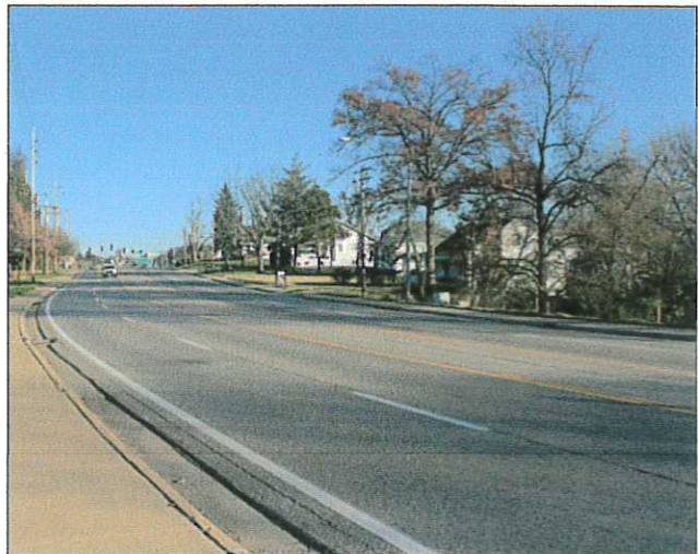
EAST OLIVE CORRIDOR
