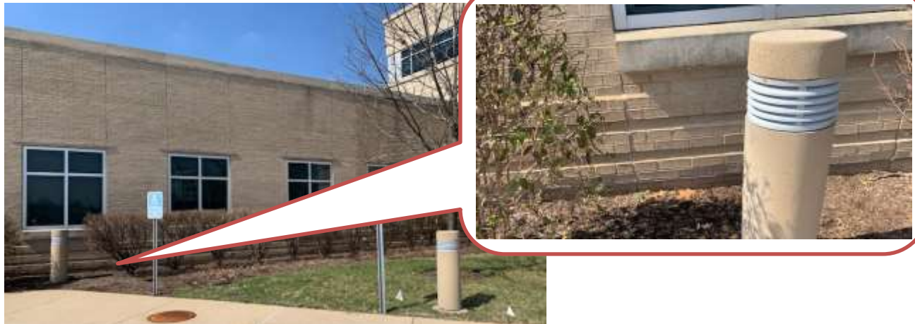
Figure 9: Close-up of the existing building with the brick relief banding along the base.
