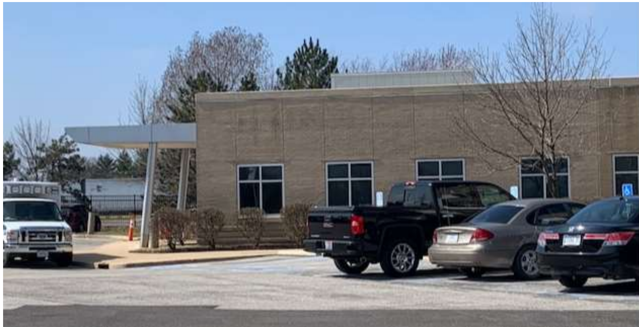
Figure 11: Photo of the existing south portion of the building showing the existing mechanical screening on the roof.
