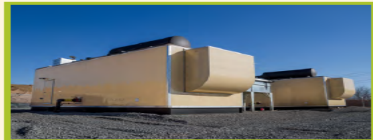
Non-recyclable trash residue from the MRF is sent to American Environmental Landfill where methane gas is captured from decomposing waste. This methane gas powers generators delivering electricity to a power plant serving a nearby community of 20,000 people.
