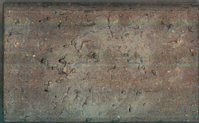
Interstate Brick - Building/Canopy Columns
