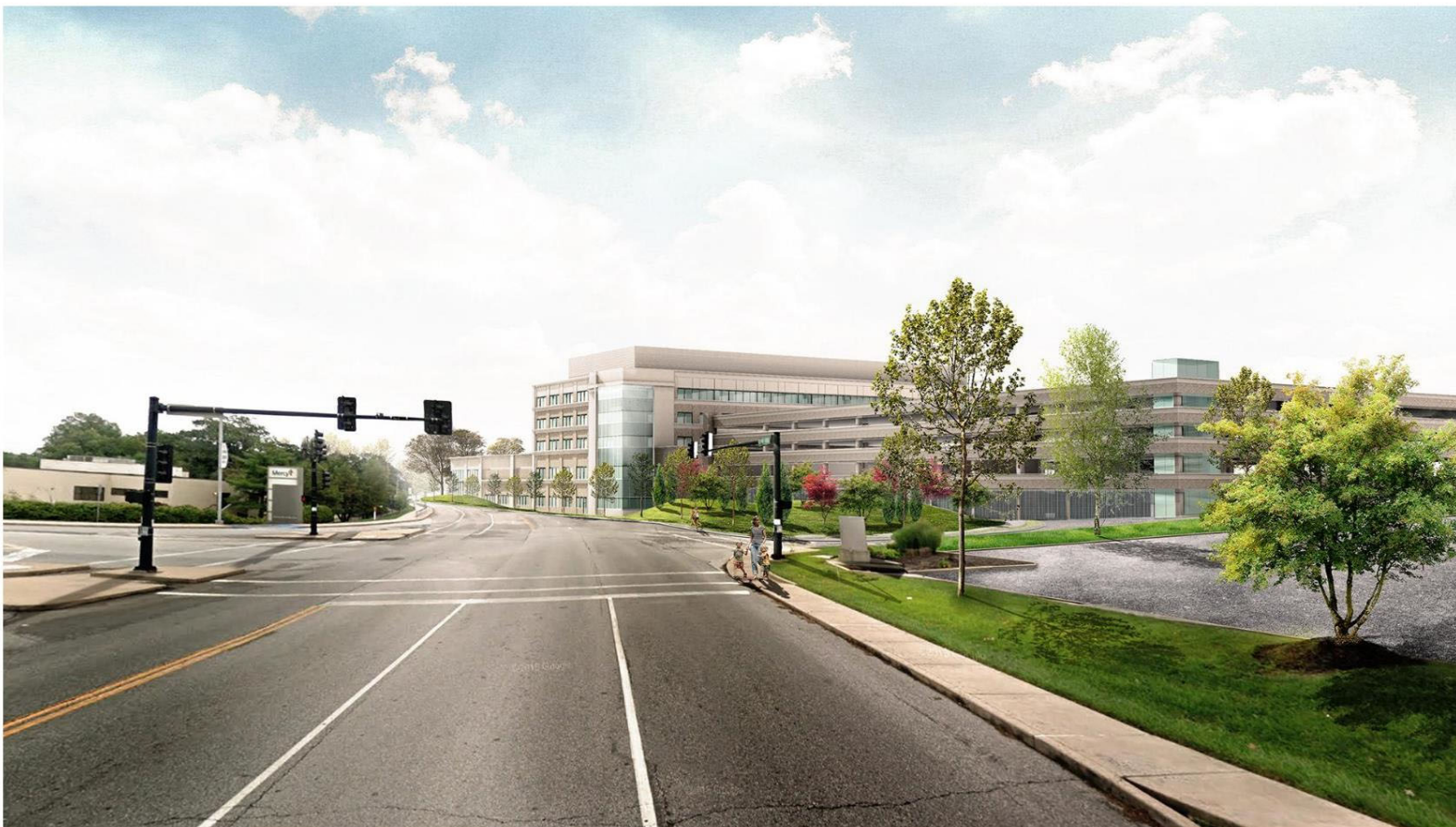
View of North side of building and parking (from eastbound Conway Rd, before Entrance Dr)
