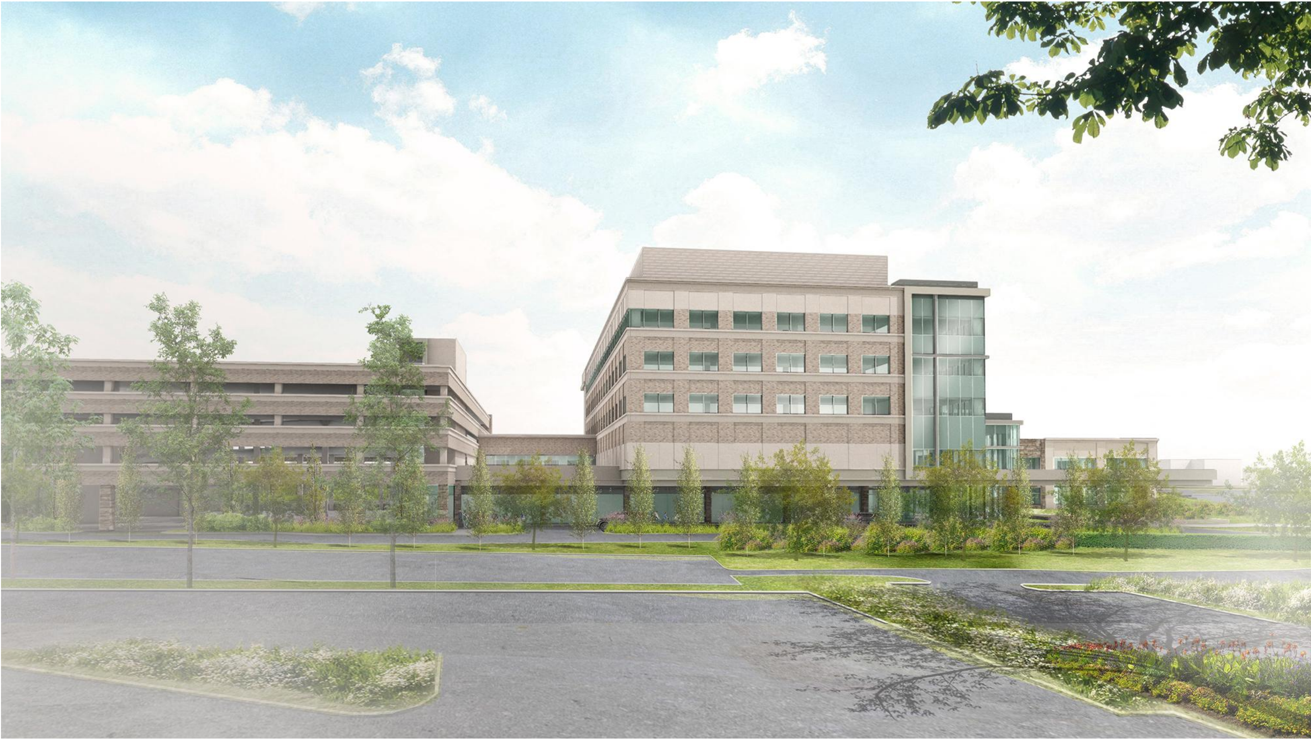
View of entry (from South, looking North)
