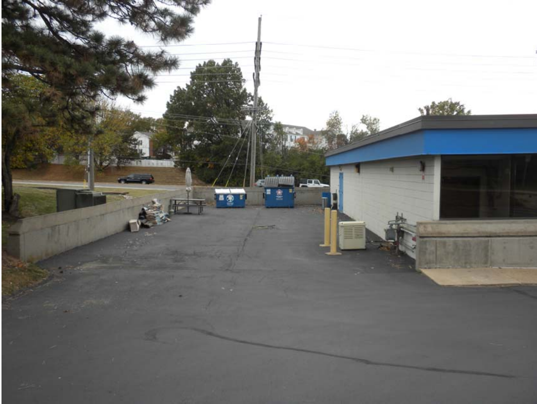
10880 BAUR BOULEVARD—SOUTH ELEVATION
