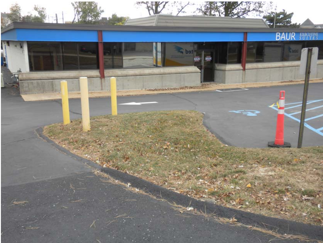
10880 BAUR BOULEVARD—EAST ELEVATION (PARTIAL)
