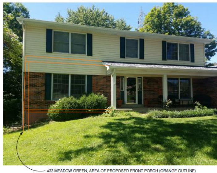
Figure 5: Applicant's images of the existing deck and front of the home.
