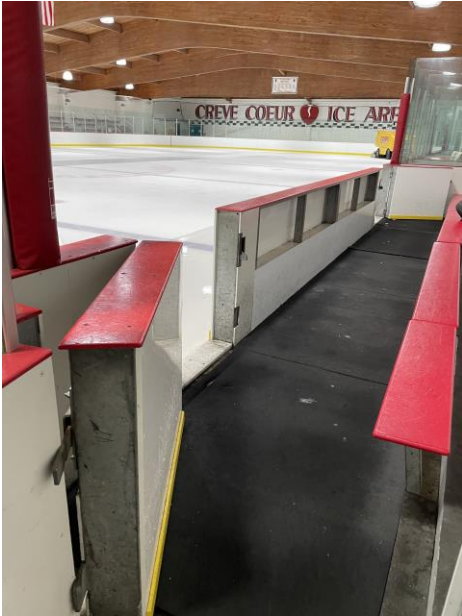
Photo 7 – Existing dasher board system
