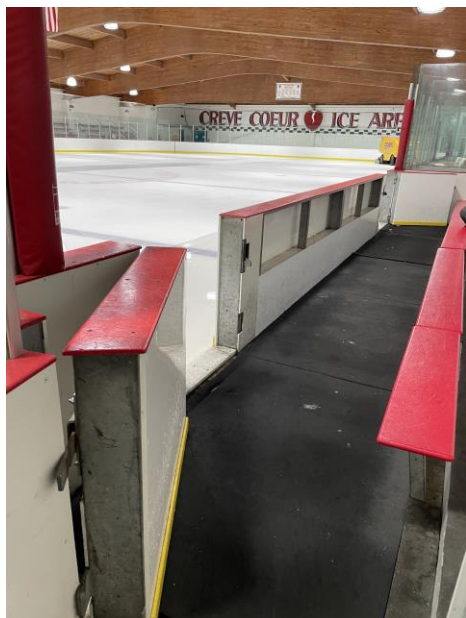
Photo 7 – Existing dasher board system
