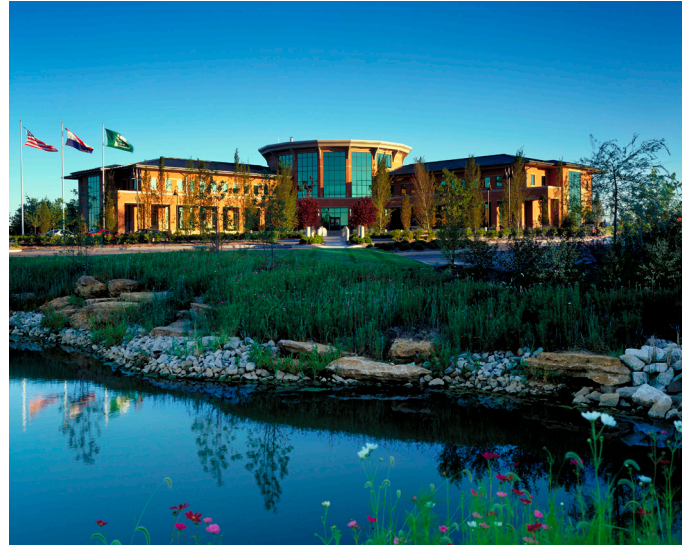
Chesterfield Government Center - Exterior landscape features utilize onsite stormwater retention basins and bedrock from excavation.
