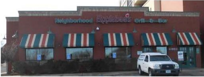
Figure 1: Prior Awnings on North Elevation
