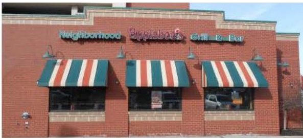
Figure 3: Prior Awnings on East Elevations
