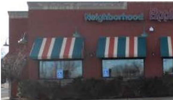
Figure 3: Close-up for prior light fixture
