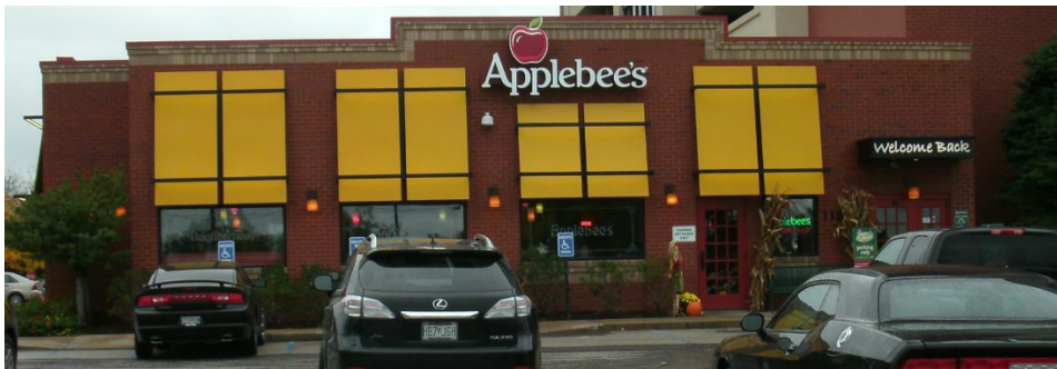
Figure 2: New Awnings and Light Fixtures on North Elevation
