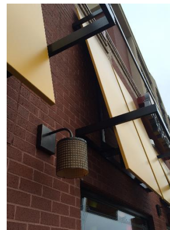
Figure 4: Close-up of new light fixtures
