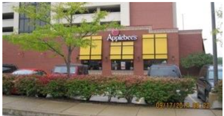
Figure 2: New Awnings and Light Fixtures on East Elevation
