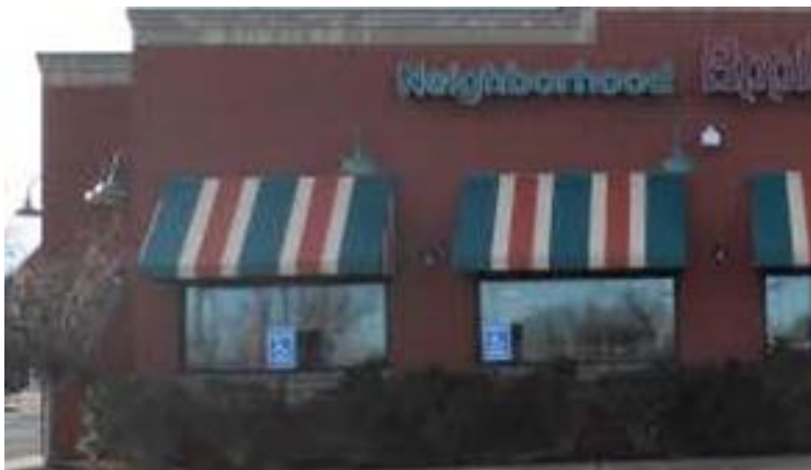
Figure 3: Close-up for prior light fixture
