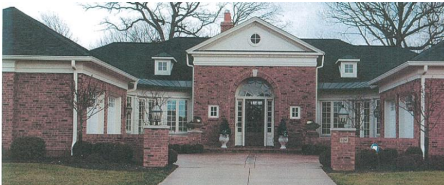
Figure 1: Photo of exiting home within the subdivision
