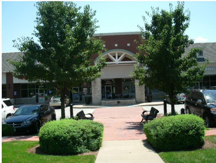
Figure 1: Photo of existing entrance
