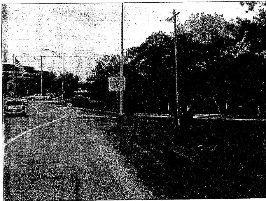
Figure 1: Eastern view of the site's frontage along Olive Boulevard.
