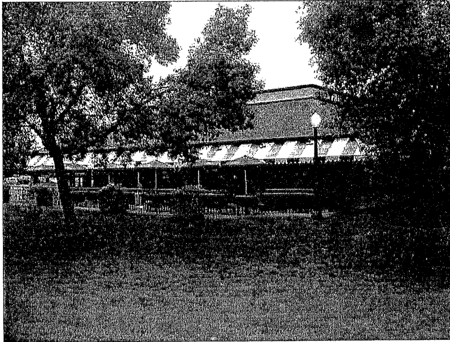
Figure 2: T.G.I. Friday's, located directly east of the subject site.
