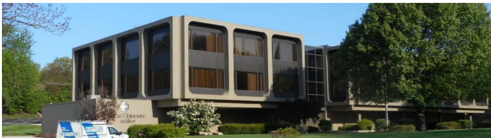
Figure 1: Close-up of the existing building. Note that the entrance is located in the middle
