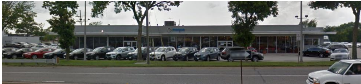
Figure 1: Google Image of the existing building.
