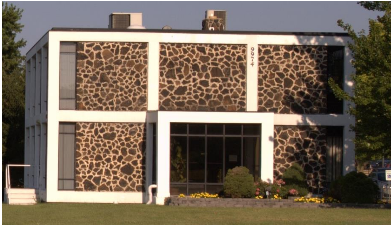
Figure 1: Existing Building (photo taken in 2013)
