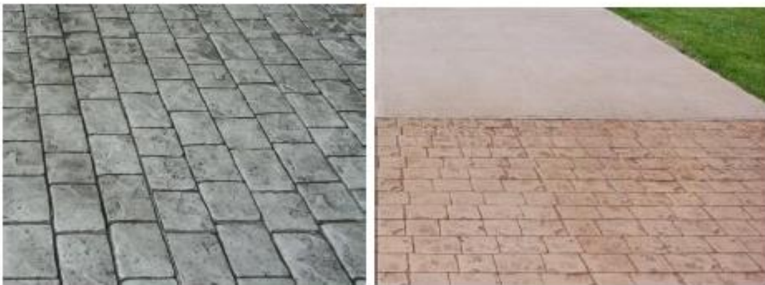
Figure 15: Close up of the Stamped concrete example from Applicant's materials.
