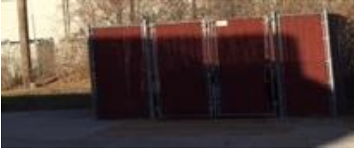
Figure 1: Close-up of the site photos showing the existing trash enclosure.
