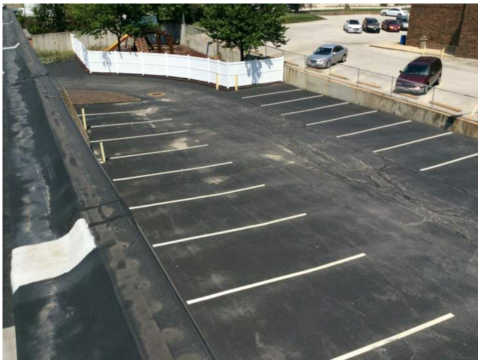
EXISTING NORTH PARKING
