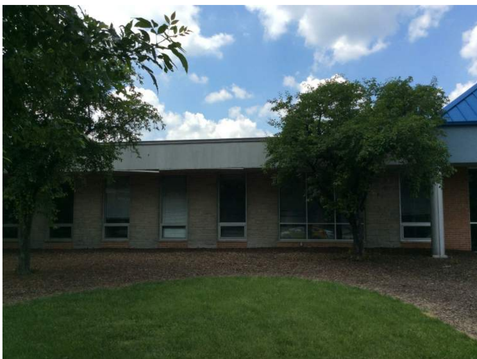
EXISTING EAST FACADE
