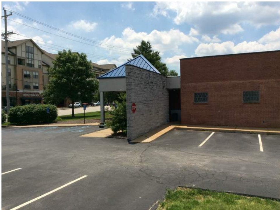
EXISTING NORTH FACADE
