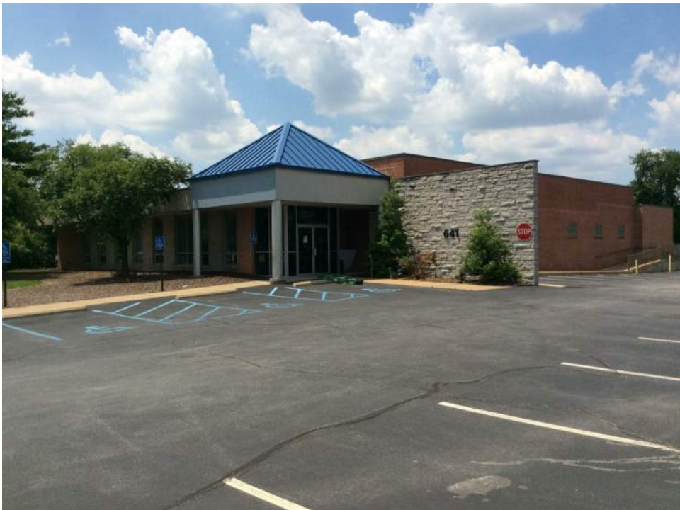
EXISTING NORTH/EAST FACADE
