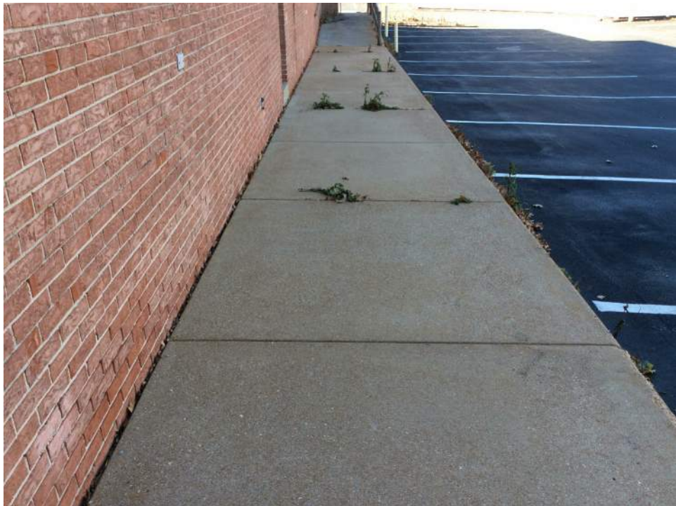
EXISTING NORTH SIDEWALK
