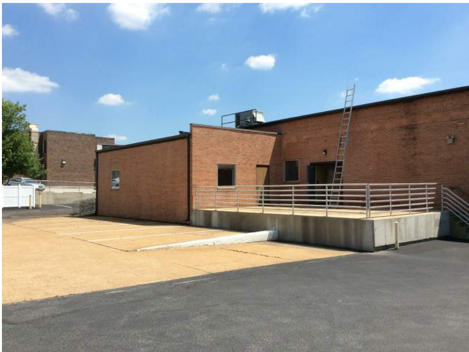
EXISTING WEST FACADE
