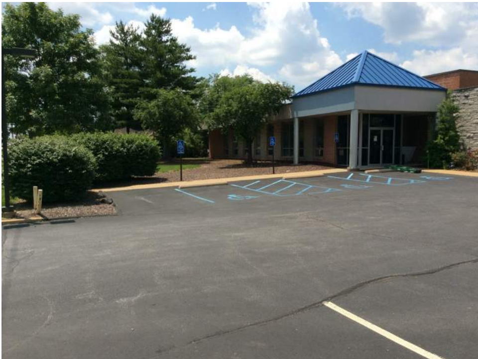
EXISTING FRONT ENTRY
