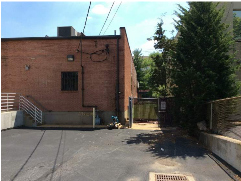
EXISTING WEST FACADE
