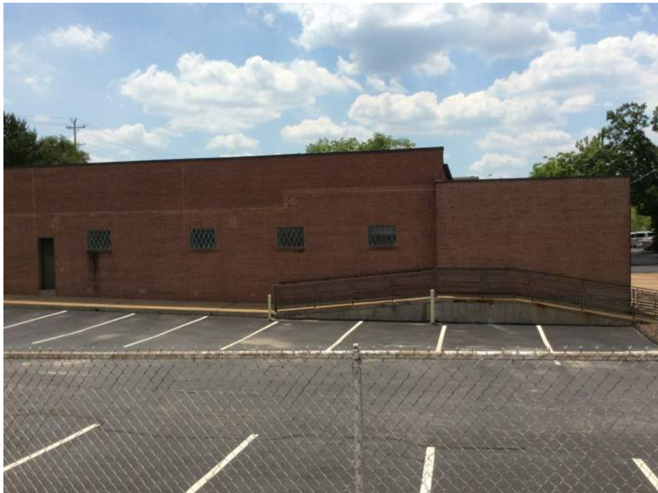
EXISTING NORTH FACADE
