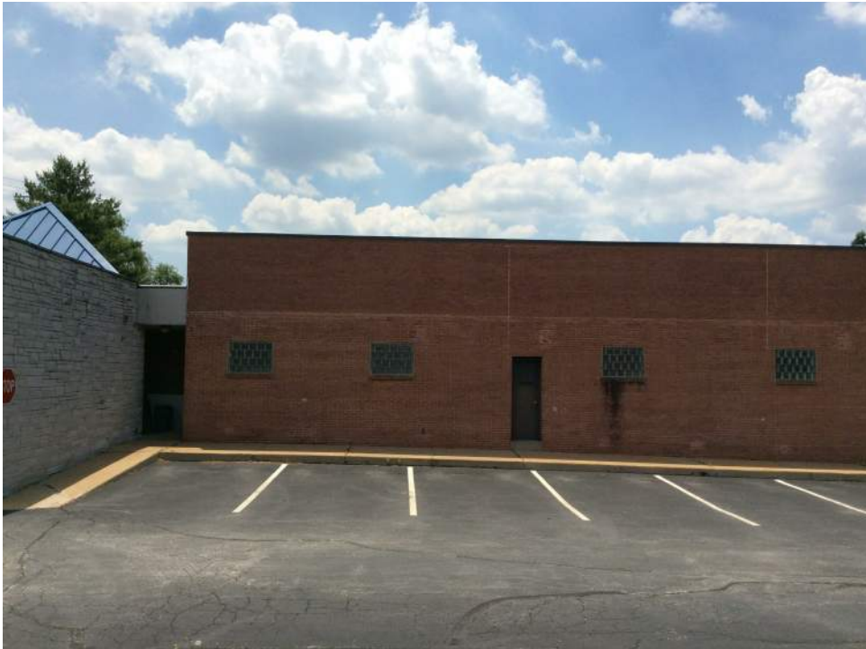
EXISTING NORTH FACADE
