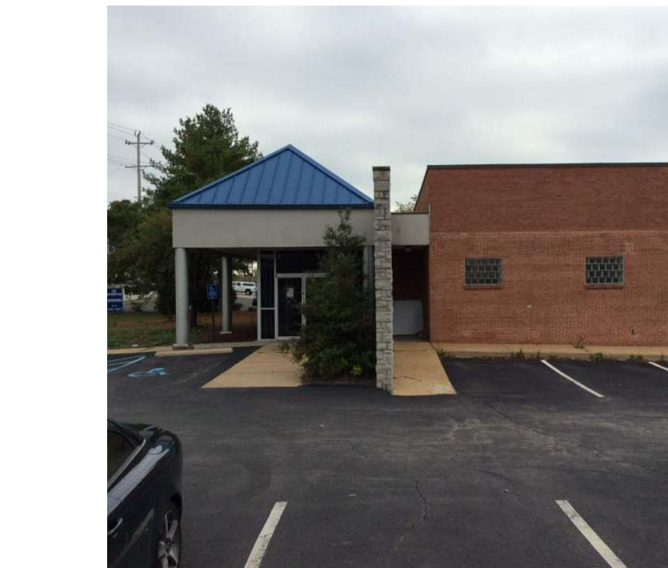
EXISTING NORTH ENTRY ELEVATION
