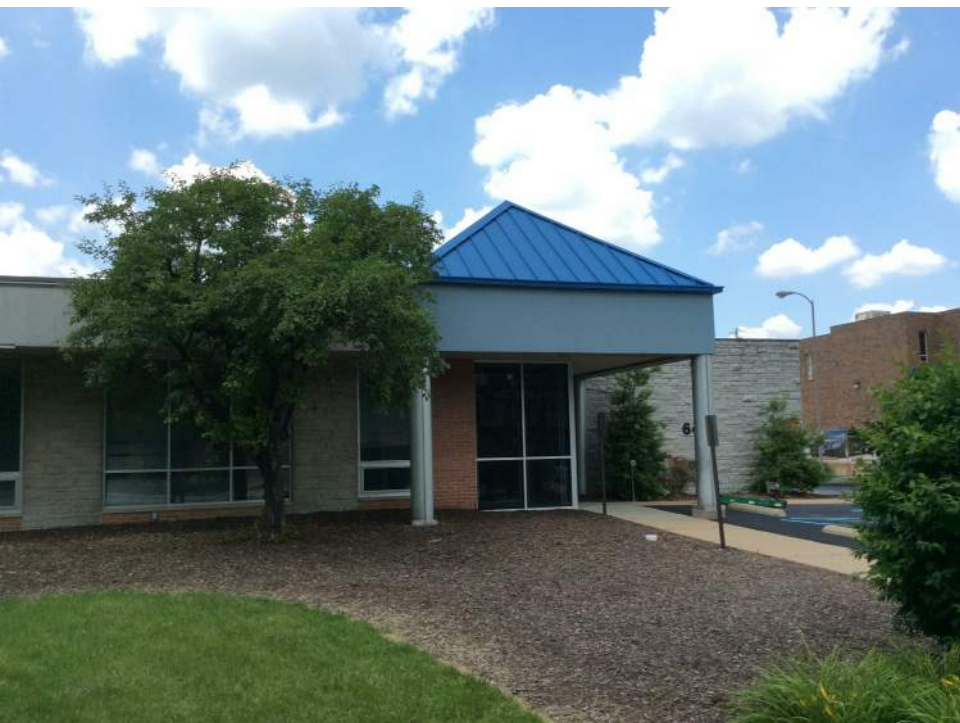
EXISTING EAST FACADE/ENTRY ELEMENT
