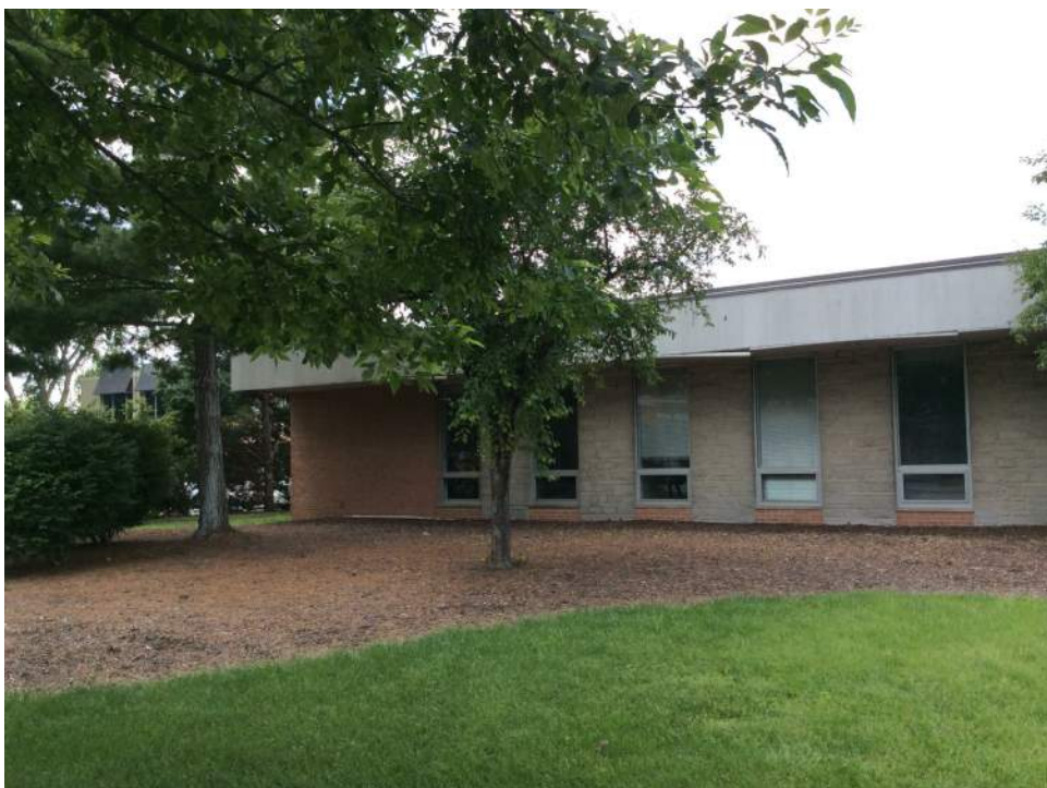
EXISTING EAST FACADE
