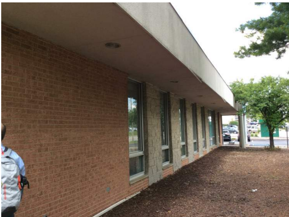
EXISTING EAST FACADE
