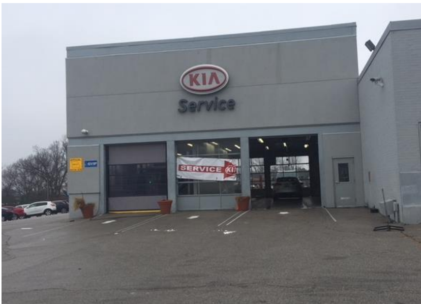
Figure 14: Photo of the existing sign of the South Elevation of the Kia Building.
