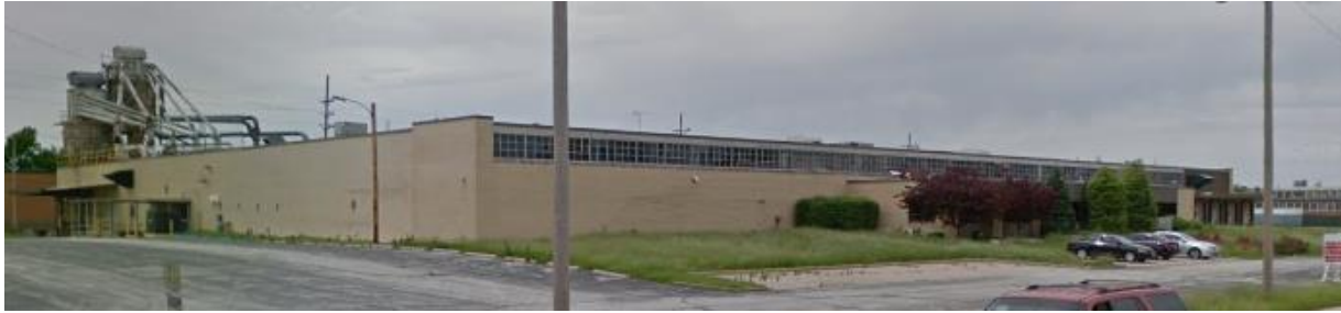
Figure 6: Google Image of the building to the south that has a brick front, and painted CMU for the larger work/warehouse area.
