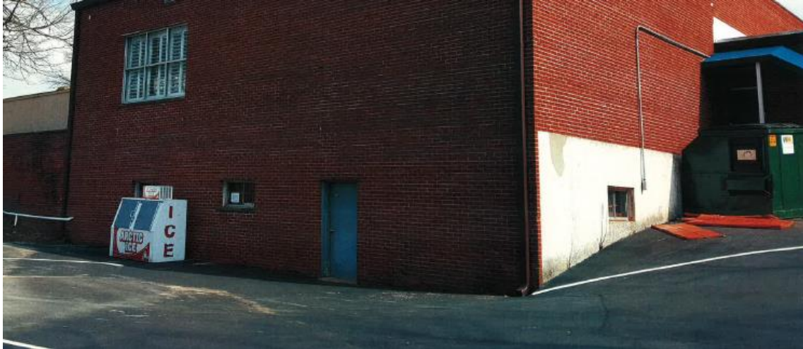
Figure 5: Close-up of the rear of the existing building showing the existing ice machine, and dumpster to the right of the photo.
