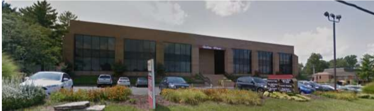
Figure 5: Google Image of the Existing Building
