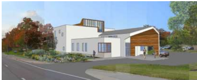
Figure 4: Rendering of the building at 227 N. Lindbergh as viewed looking south along Lindbergh Boulevard, from the 2012 renovation of the office building.
