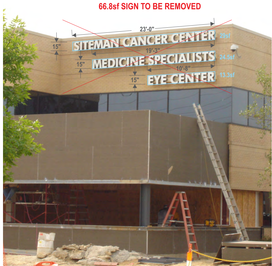
EXISTING CHANNEL LETTER SIGN TO BE REMOVED
