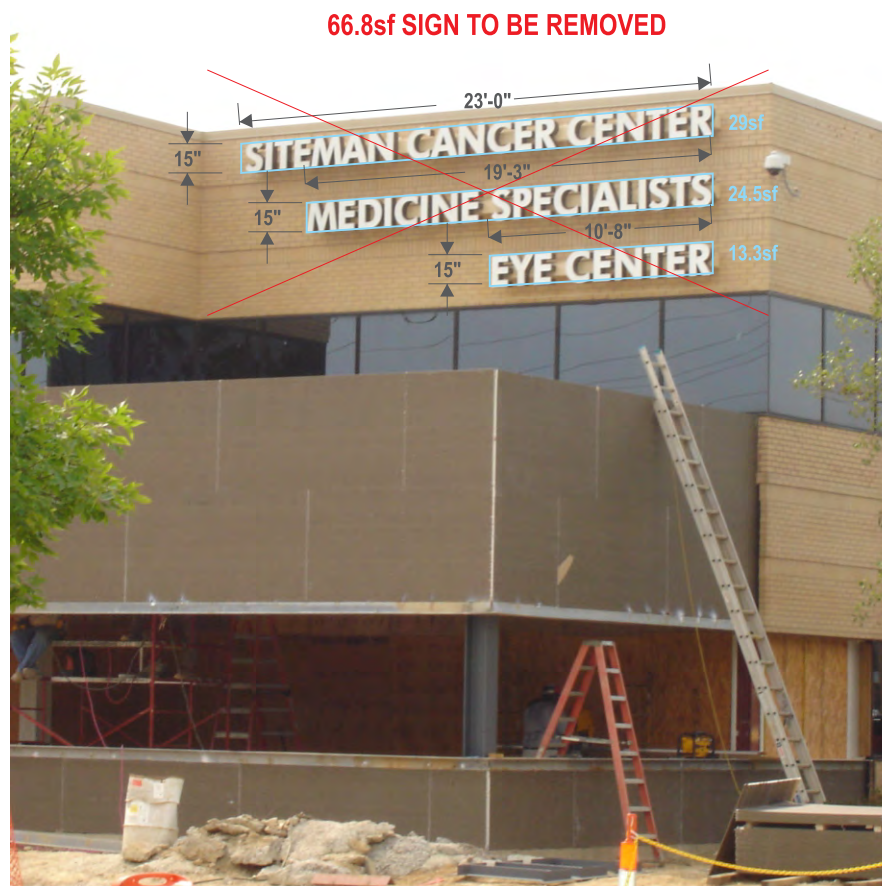
EXISTING CHANNEL LETTER SIGN TO BE REMOVED
