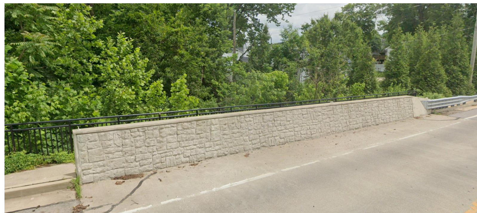
Standard Concrete Hanna Road, Manchester
