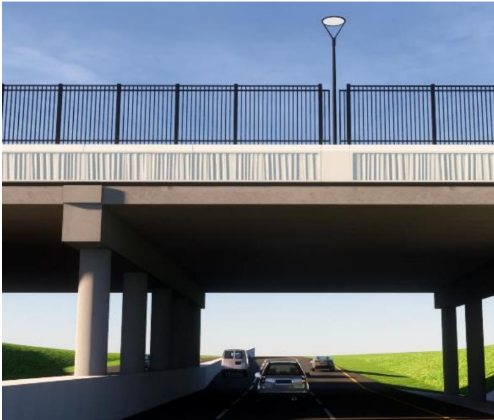
Image 3: Revised formliner bridge face design
