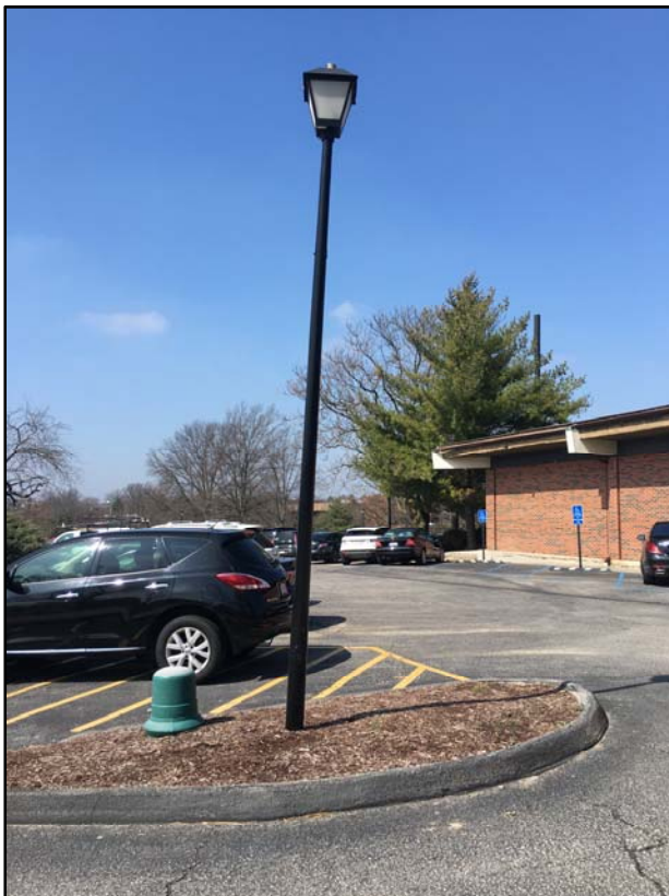
Figure 1. Existing post-top light in the western Dielmann Recreation Complex parking lot.
