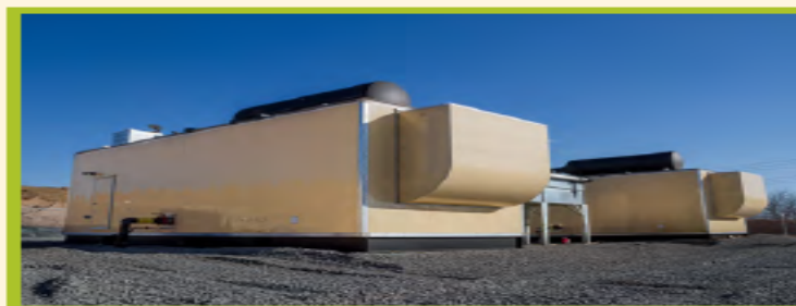
Non-recyclable trash residue from the MRF is sent to American Environmental Landfill where methane gas is captured from decomposing waste. This methane gas powers generators delivering electricity to a power plant serving a nearby community of 20,000 people.
