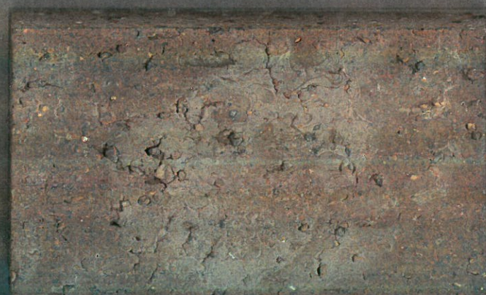
Interstate Brick - Building/Canopy Columns
