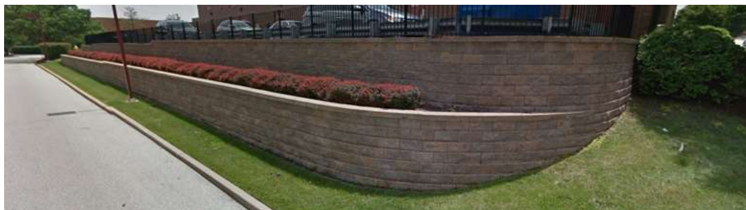
Figure 12: Google Image of the retaining wall to the south of the proposed development behind the retail center.
