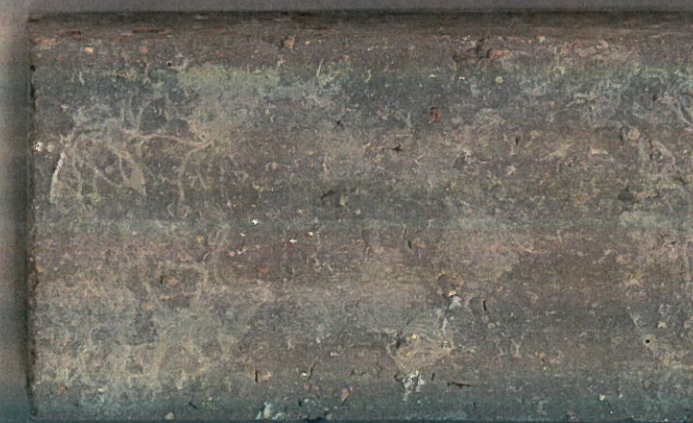
Interstate Brick - Building/Canopy Columns
