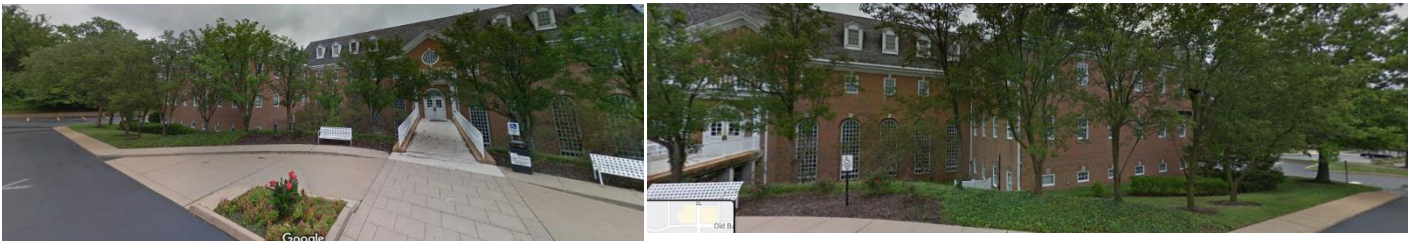
Figure 11: Google images of the prior landscaping in front of 522 N. New Ballas Road.
