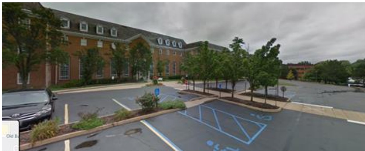
Figure 14: Google Image of the prior landscaping in front of 456 N. New Ballas Road
