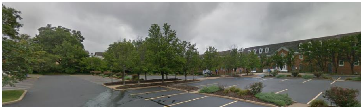
Figure 8: Google Image of the prior landscaping of the parking lot islands that have been removed
