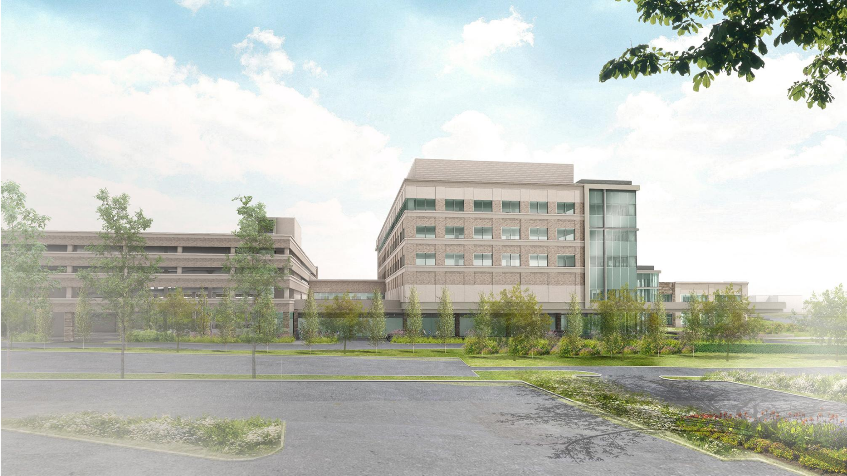
View of entry (from South, looking North)
