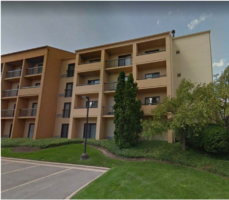
2 EXTERIOR PHOTOS - SOUTH 3/32" = 1'-0"
