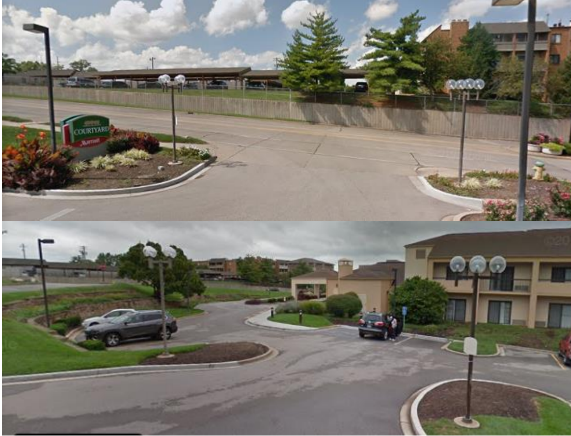
Figure 10: Google images of the non-conforming bulb lights at the entrances to the site.
