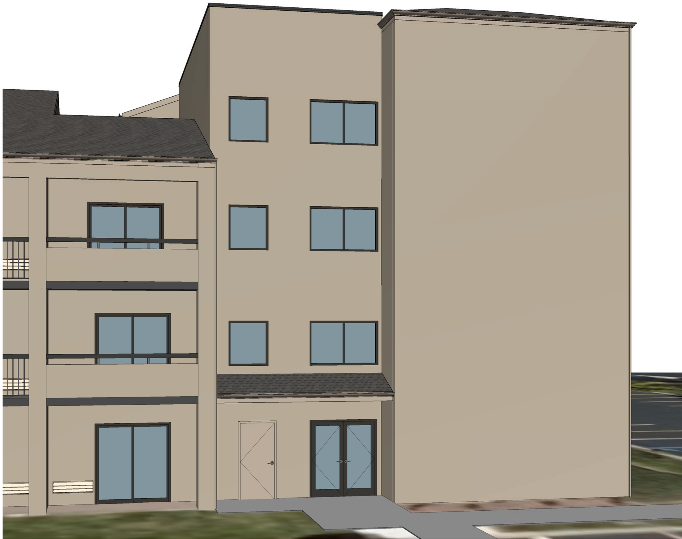
4 SOUTH REAR ENTRY - EXISTING
