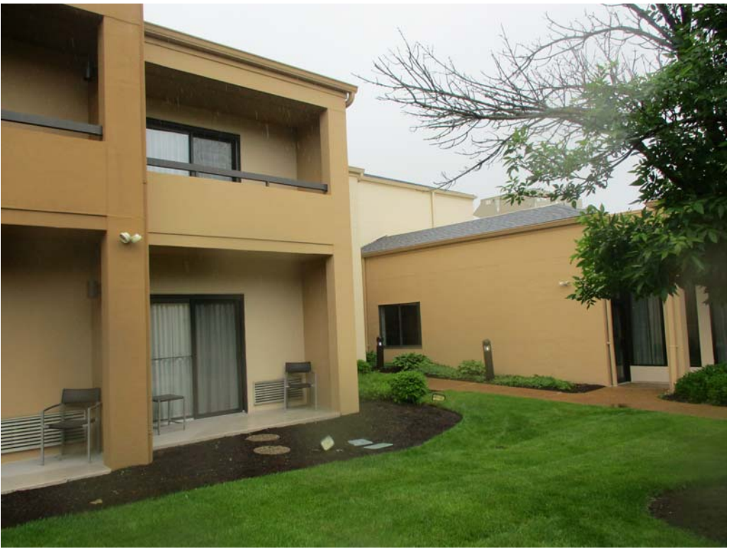
3 EXTERIOR PHOTOS - SOUTH COURTYARD 3/32" = 1'-0"
