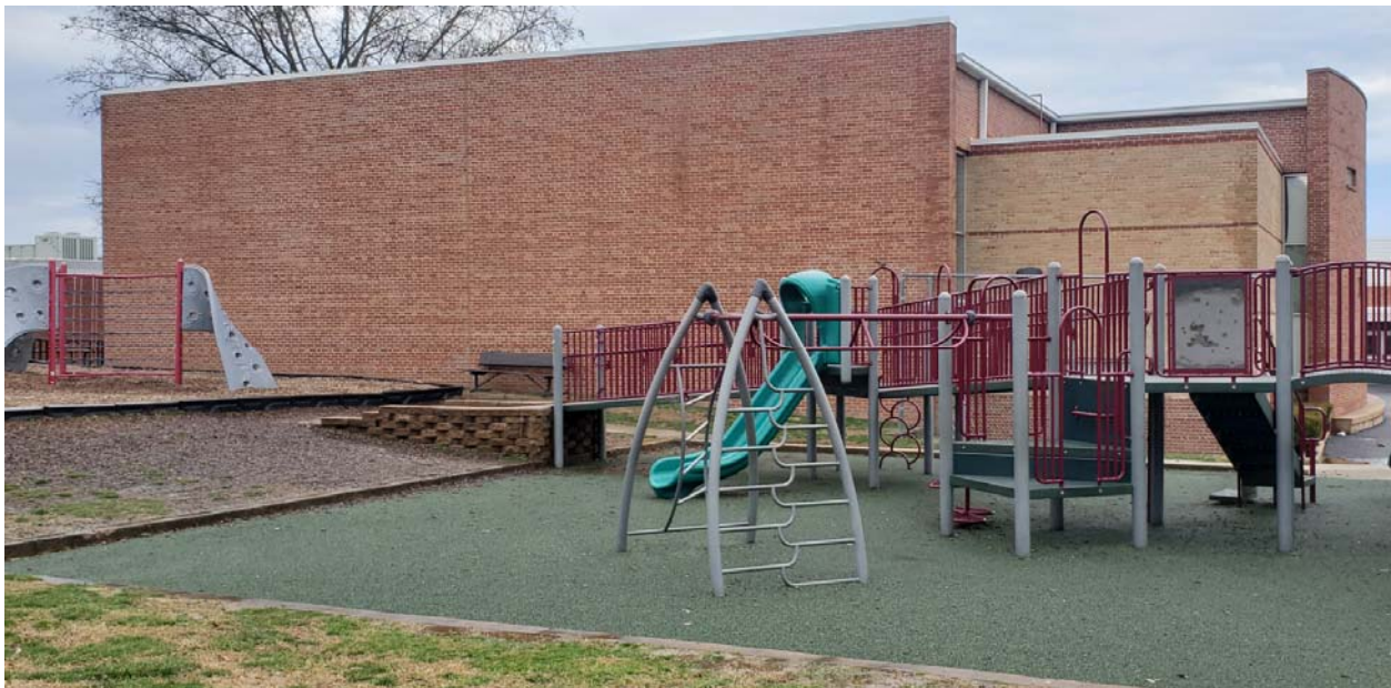
View of existing west Gym Addition elevation
