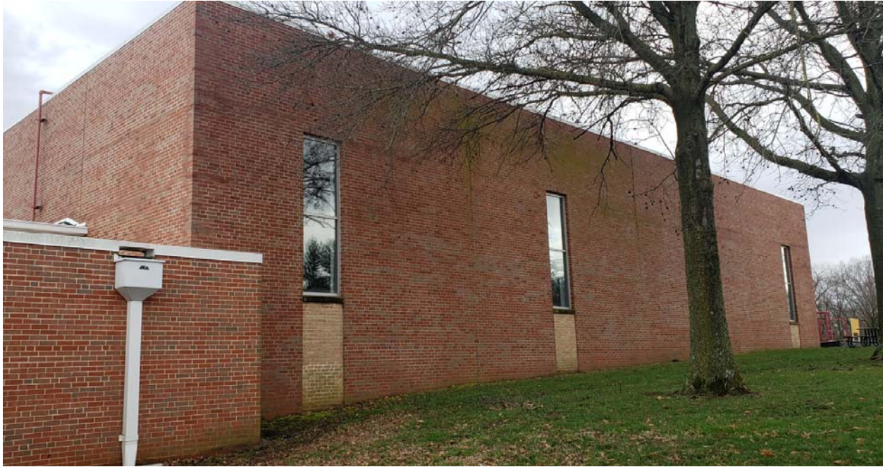
View of existing north Gym Addition elevation
