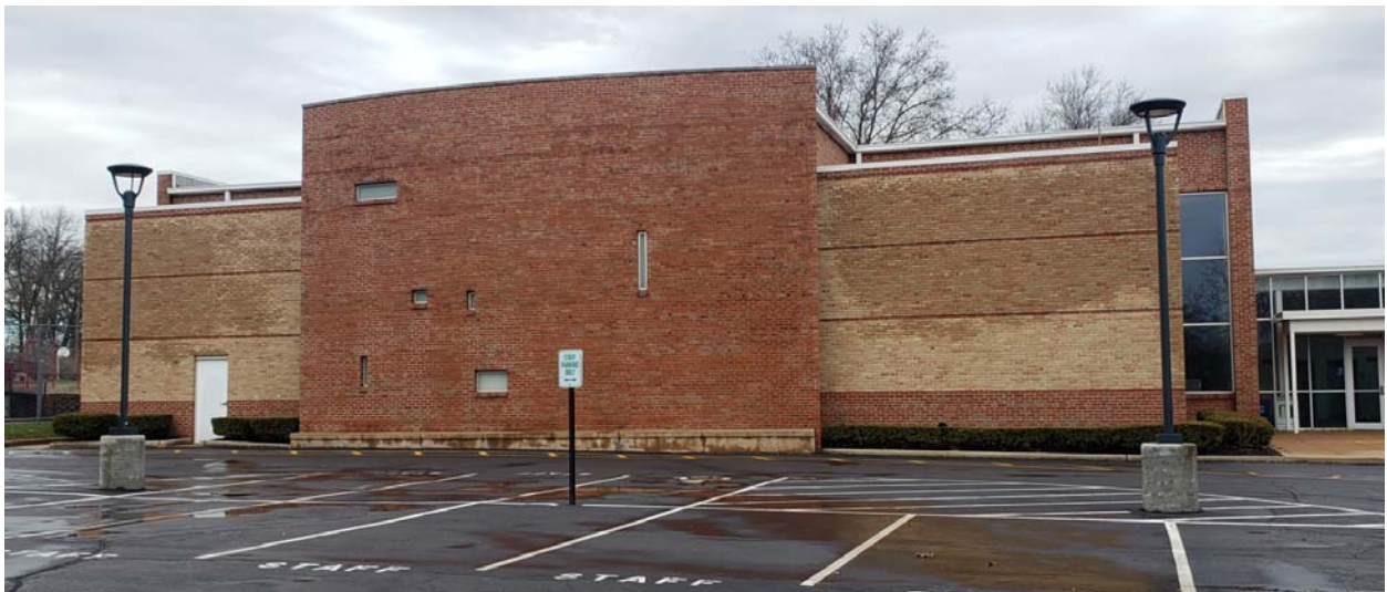
View of existing south Gym Addition elevation
