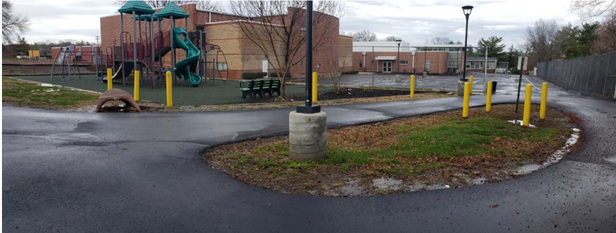
View of existing playground and Gym Addition looking north-east
