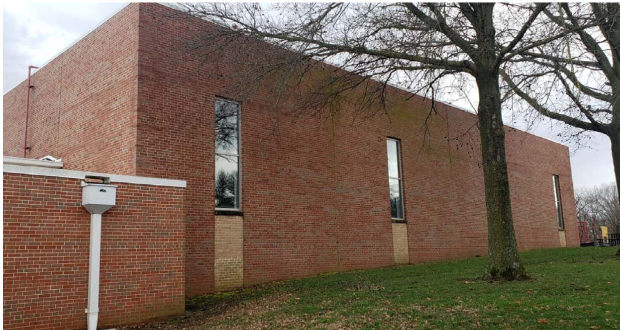
View of existing north Gym Addition elevation
