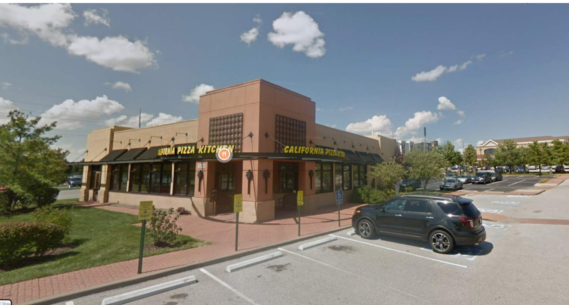
EXISTING BUILDING ON PROJECT SITE CALIFORNIA PIZZA KITCHEN
