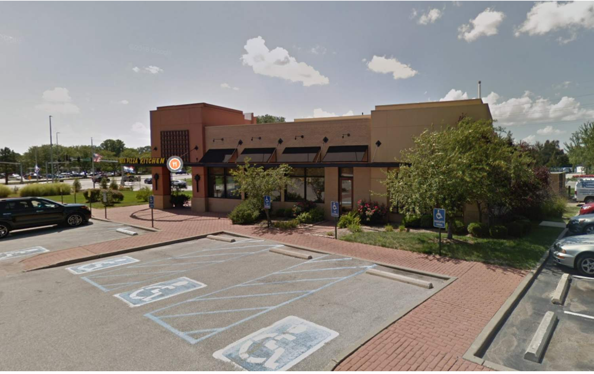
EXISTING BUILDING ON PROJECT SITE CALIFORNIA PIZZA KITCHEN
