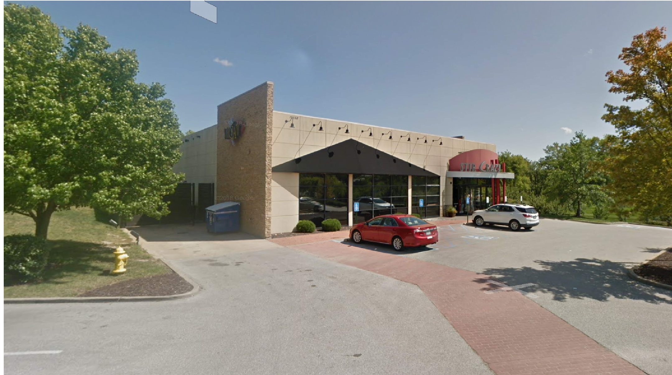
EXISTING BUILDING ON PROJECT SITE STIR CRAZY
