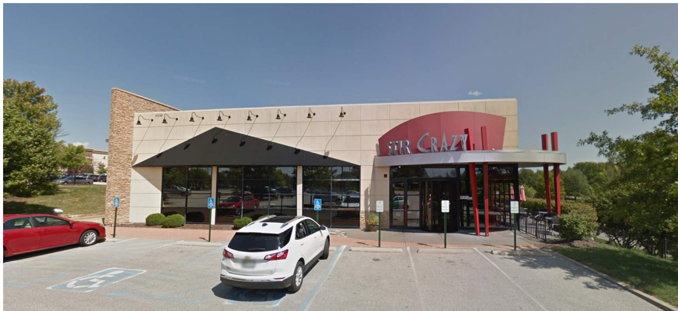
EXISTING BUILDING ON PROJECT SITE STIR CRAZY
