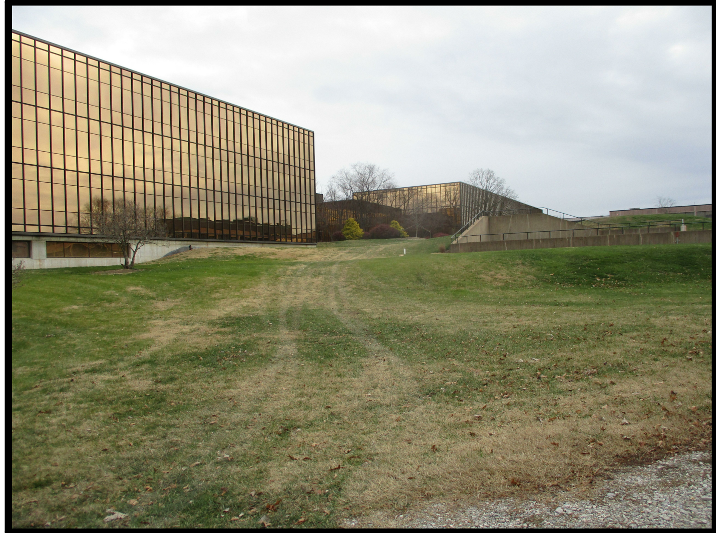
9. EXISTING BUILDING G & COURT #1
