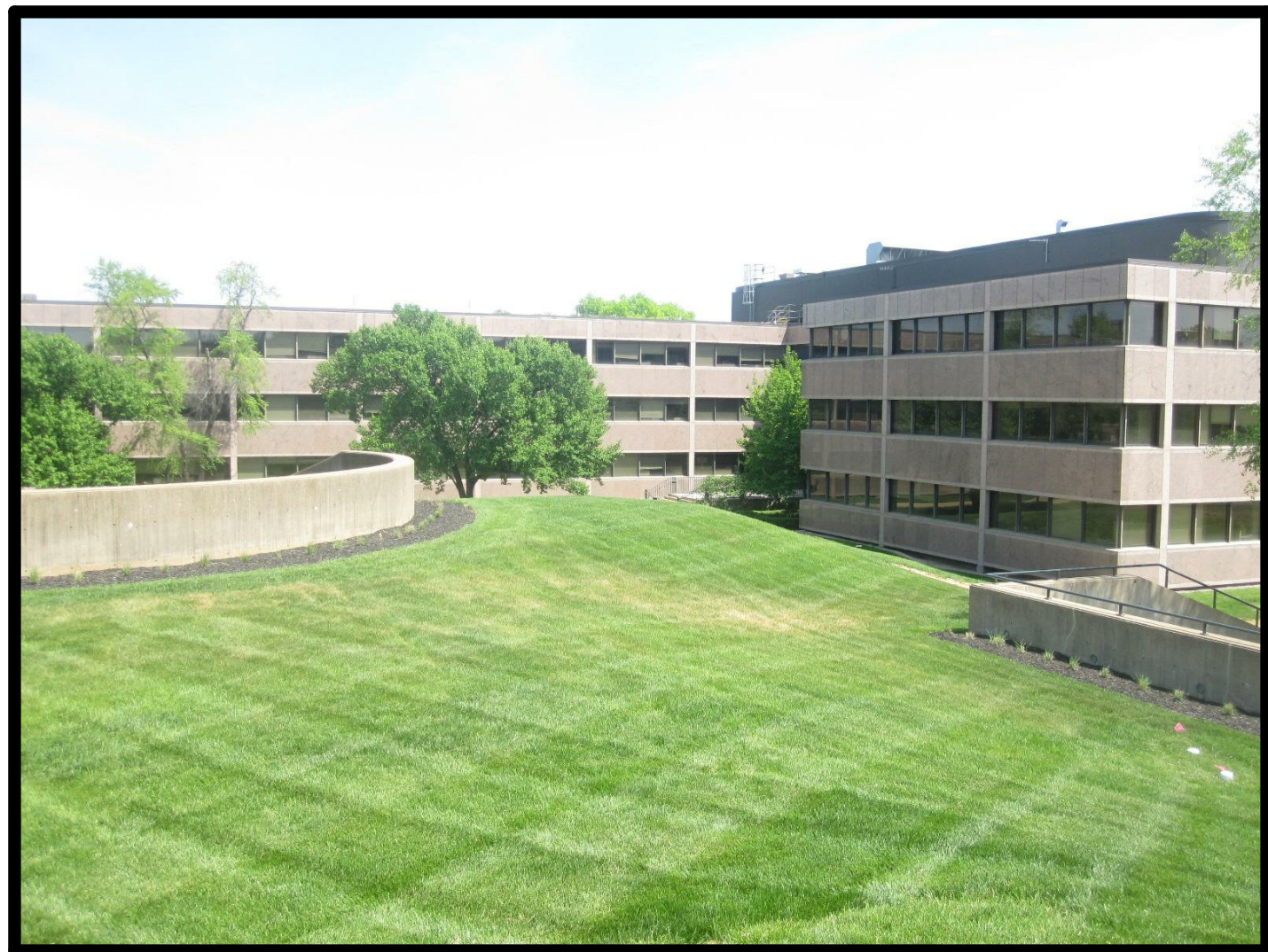
12. EXISTING BUILDING F & COURT #2 & #4
