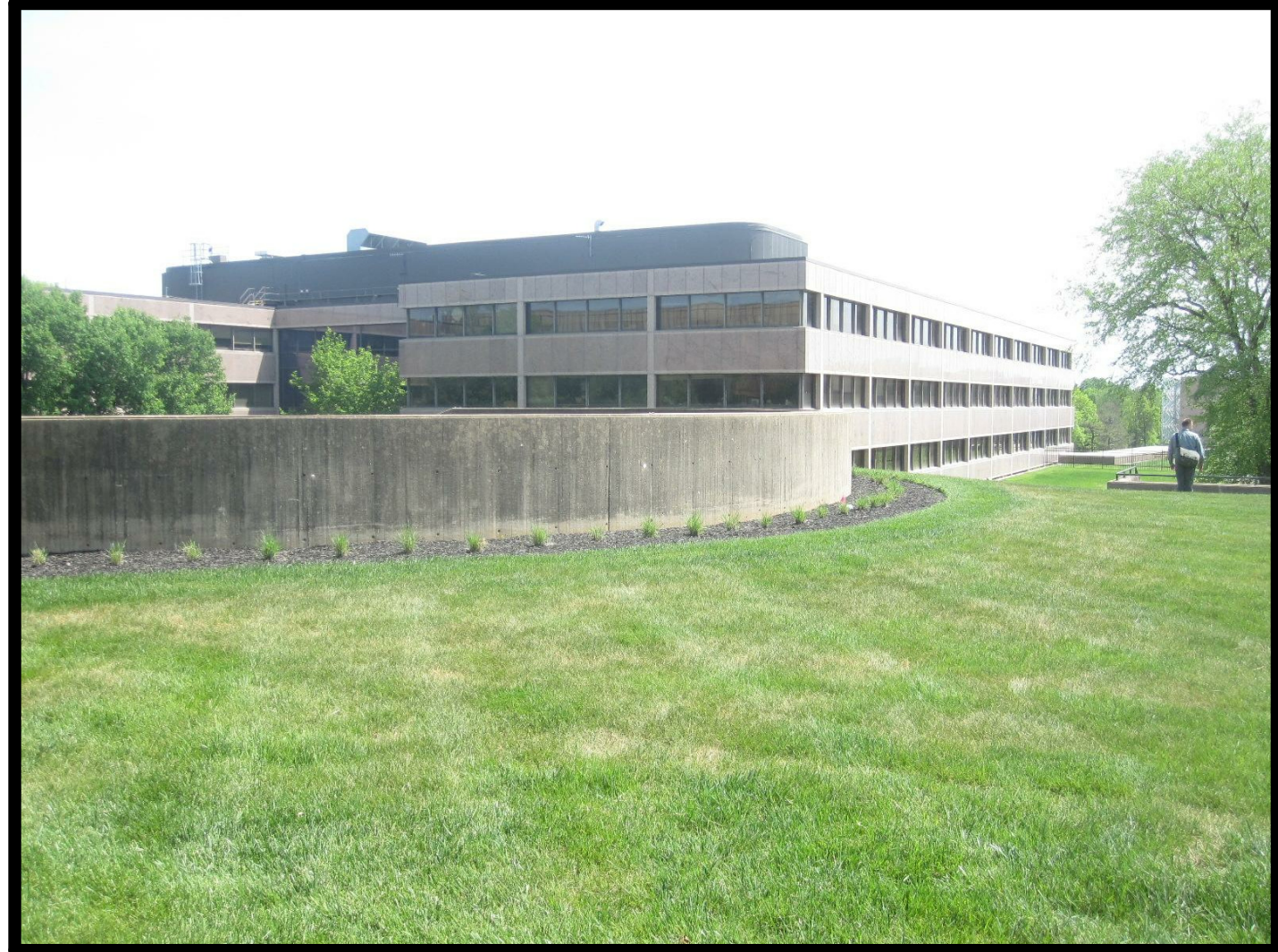
10. EXISTING BUILDING F & COURT #2
