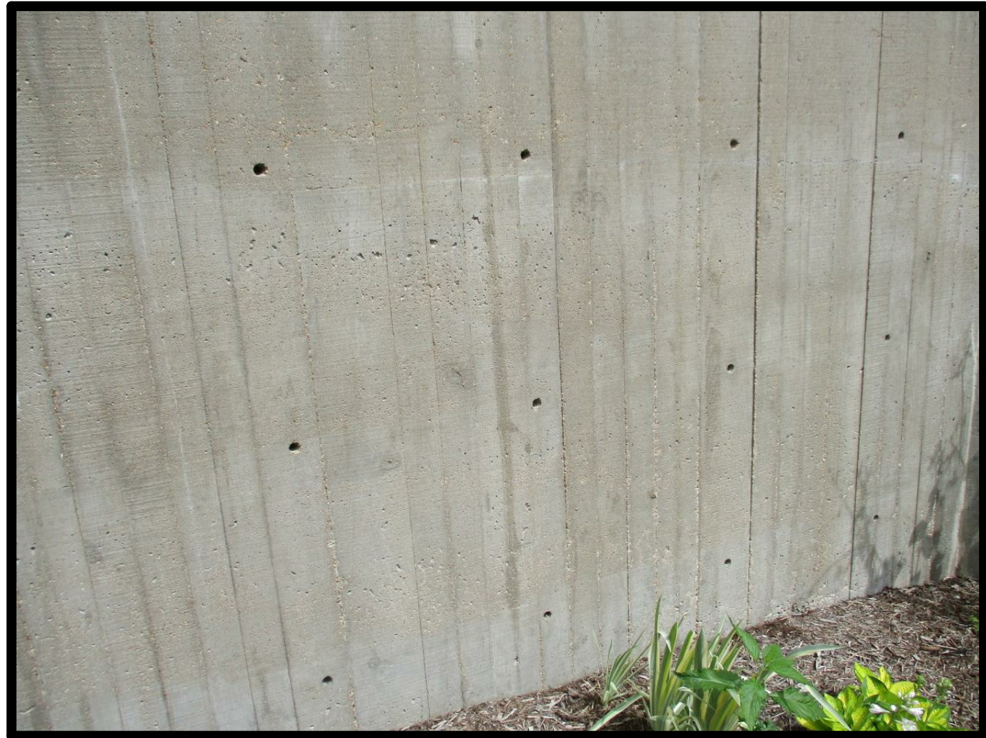
1. EXISTING TYPICAL BOARD FORMED CONCRETE WALL
