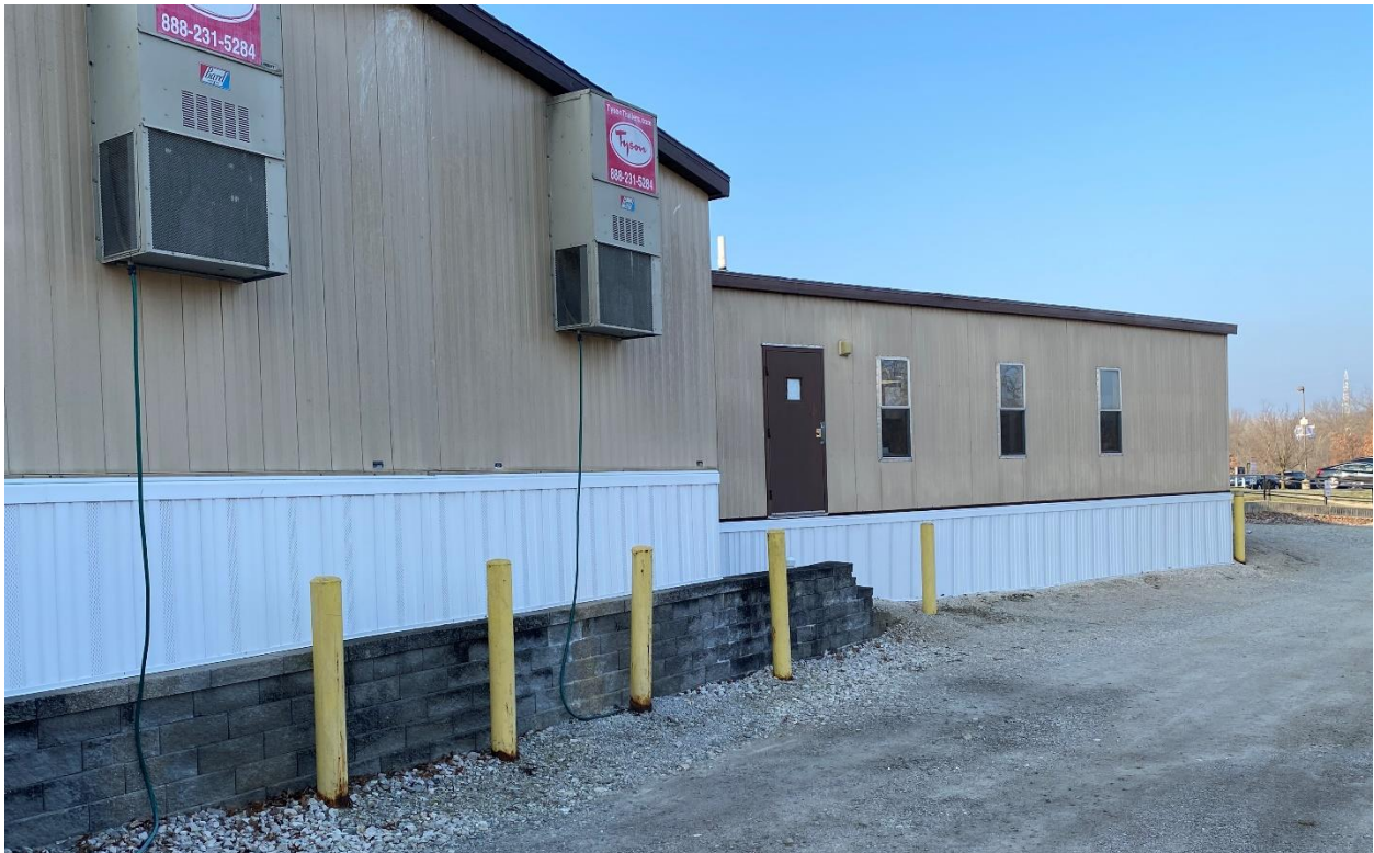
North side of modular office buildings
