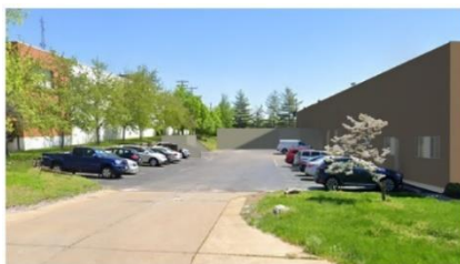
PUBLIC VIEW OF NORTH PARKING LOT, OUTDOOR MECHANICAL SCREEN WALL AND DUMPSTER ENCLOSURE
