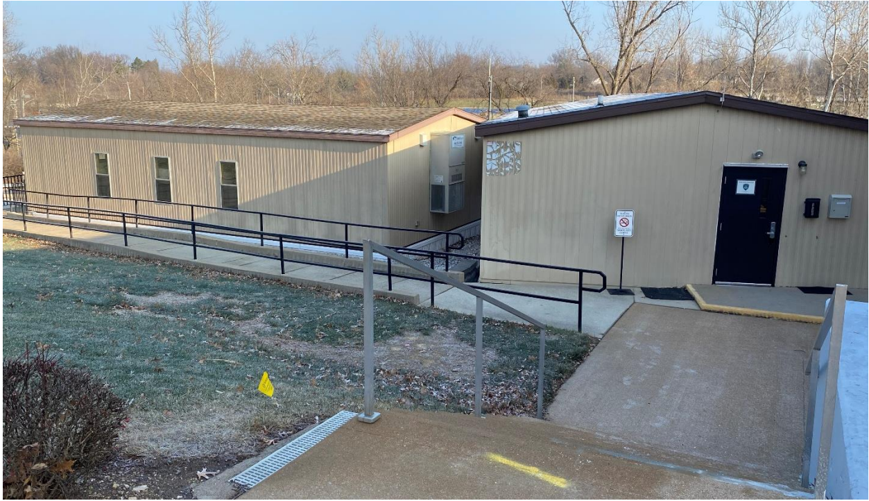
South side of modular office buildings
