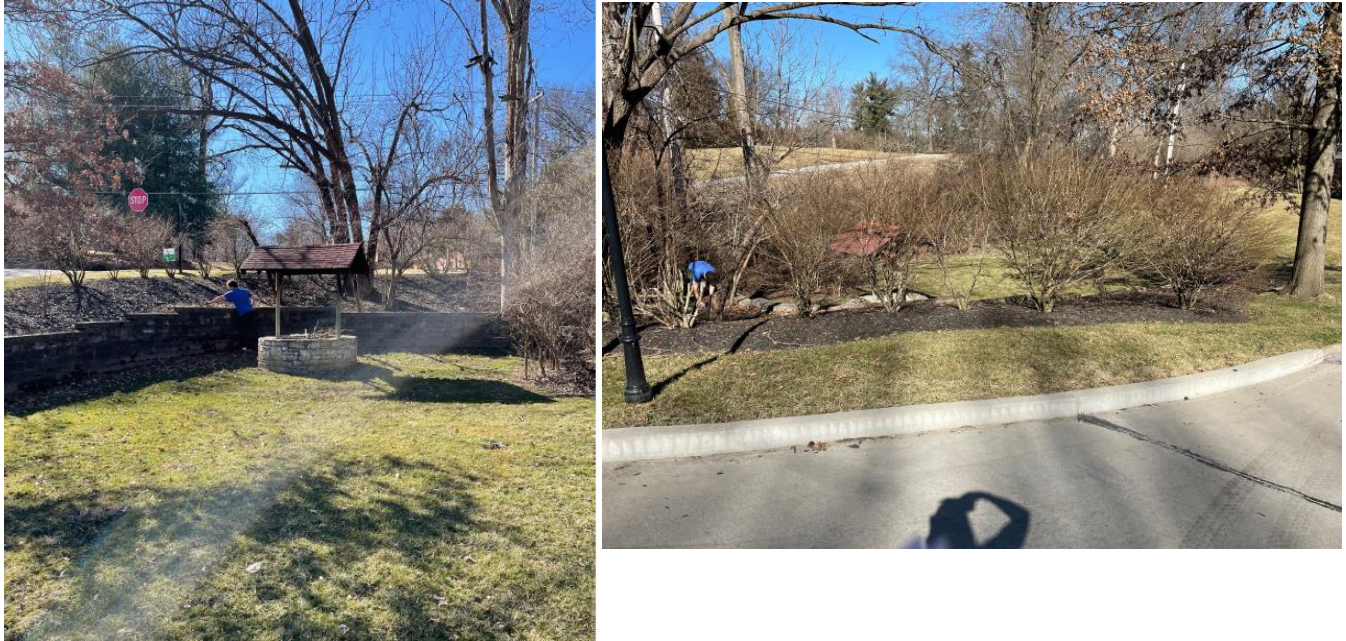
Figure 2: Applicant's photos of the existing retaining wall, and view from N. Spoede Road.
