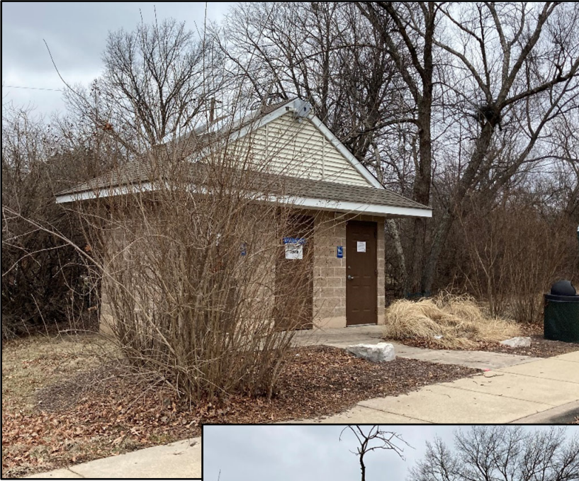
Existing Conway Park Restroom
