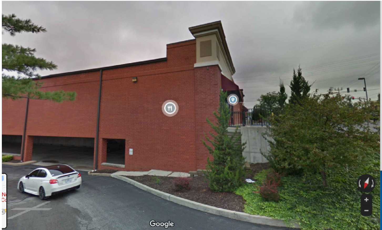
2 existing structure - north elevation
