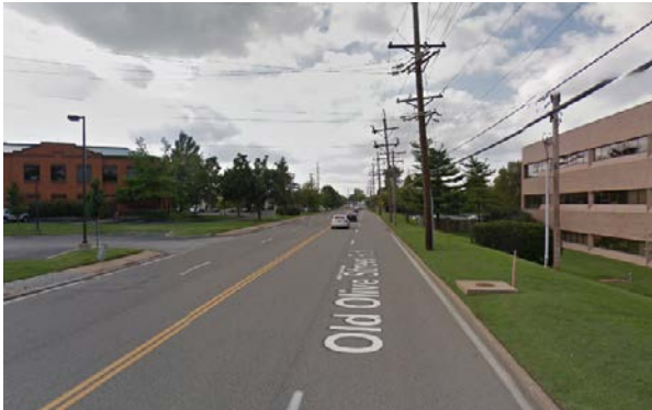
OLD OLIVE STREET ROAD
