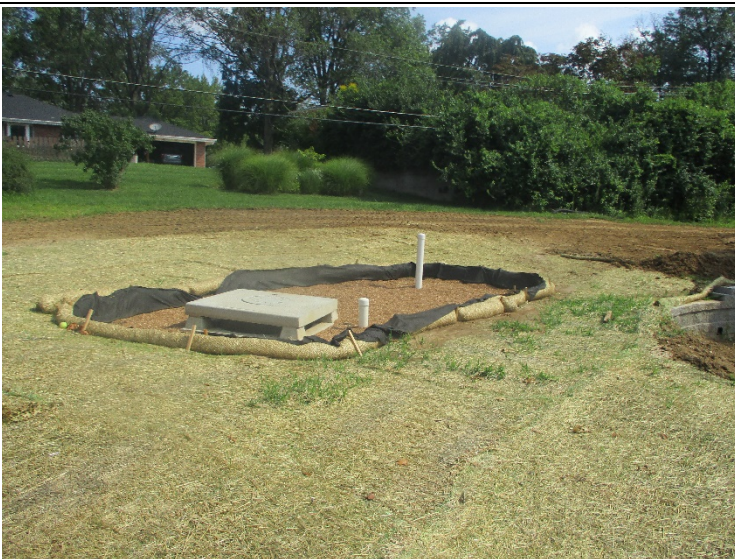
Photograph: #08 Taken By: Josh Rivers Date Taken: 8/17/2021 Program: WPC Unit Entity: City of Creve Coeur Permit: MOR040005 Location: Santino Court Description: Post construction BMP being installed. Ensure it is not affected by active development.
