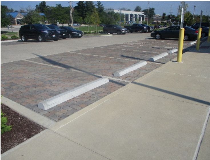
Photograph: #07 Taken By: Josh Rivers Date Taken: 8/17/2021 Program: WPC Unit Entity: City of Creve Coeur Permit: MOR040005 Location: Creve Coeur Police Station Description: Pervious pavement
