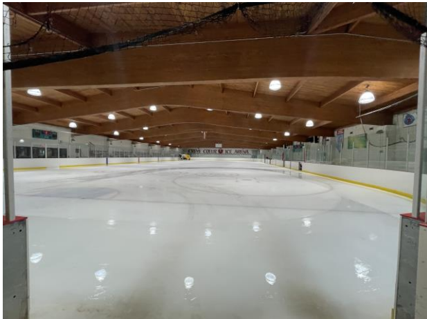
Photo 5 – Overall ice rink floor
