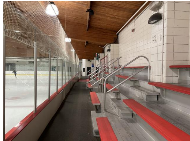
Photo 6 – Bleacher seating in ice arena
