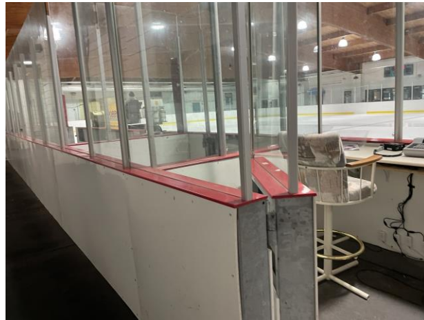
Photo 8 – Existing dasher board system – Scorer's box
