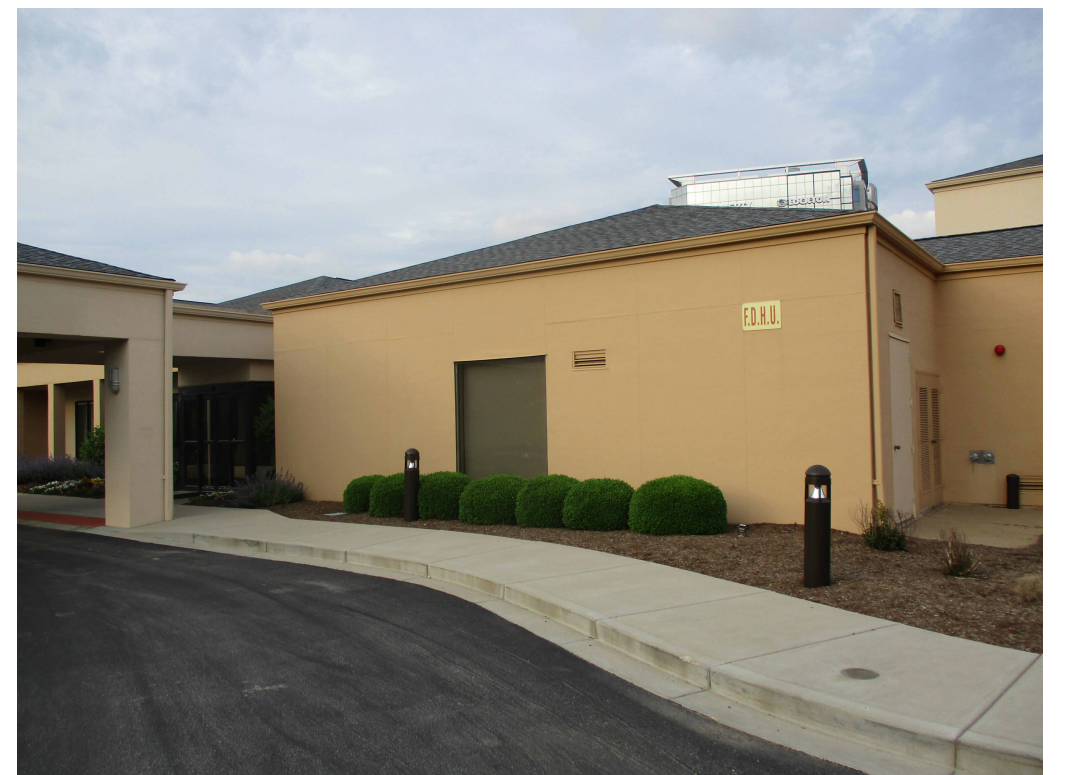
1 EXTERIOR PHOTOS - WEST 12" = 1'-0"
