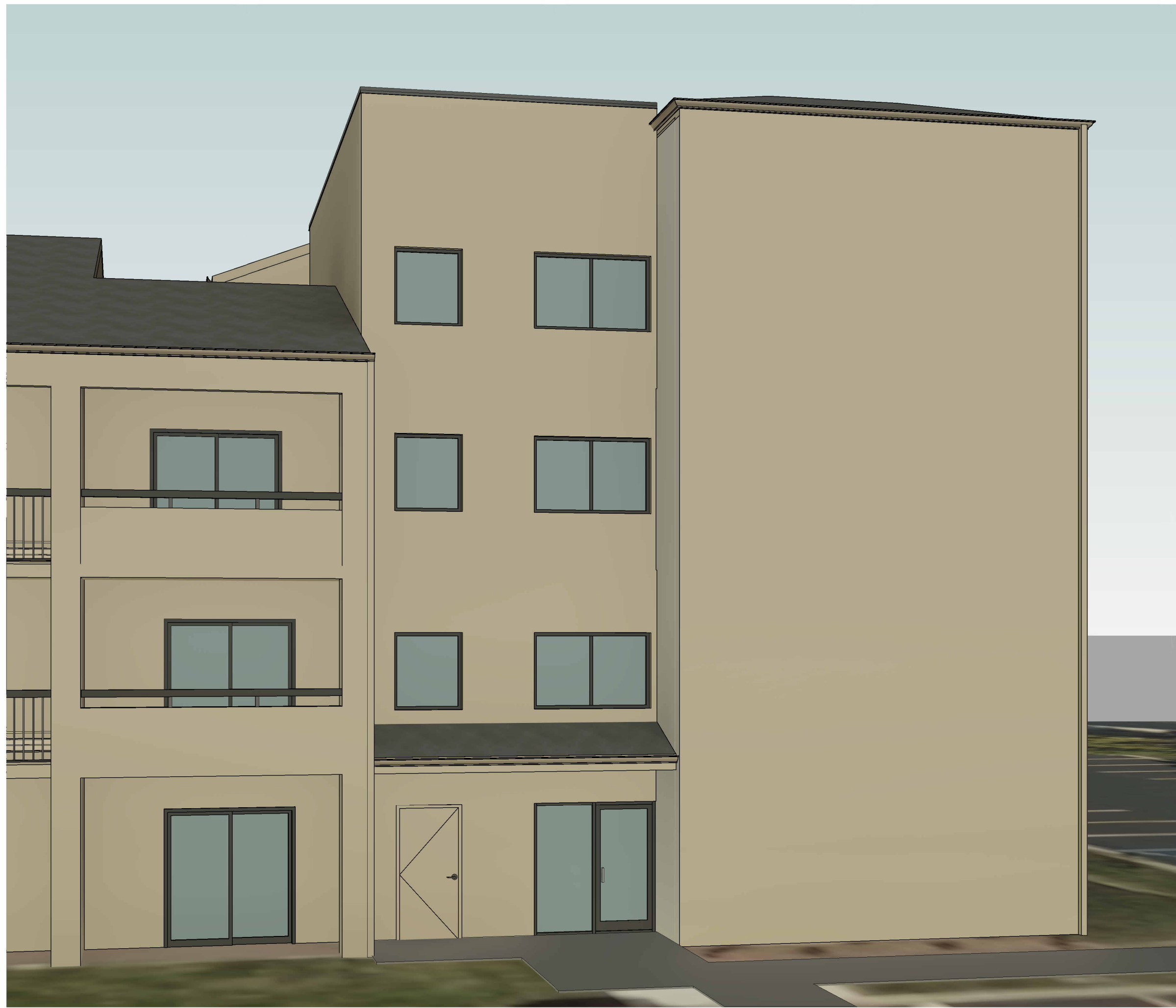
3 SOUTH REAR ENTRY - EXISTING
