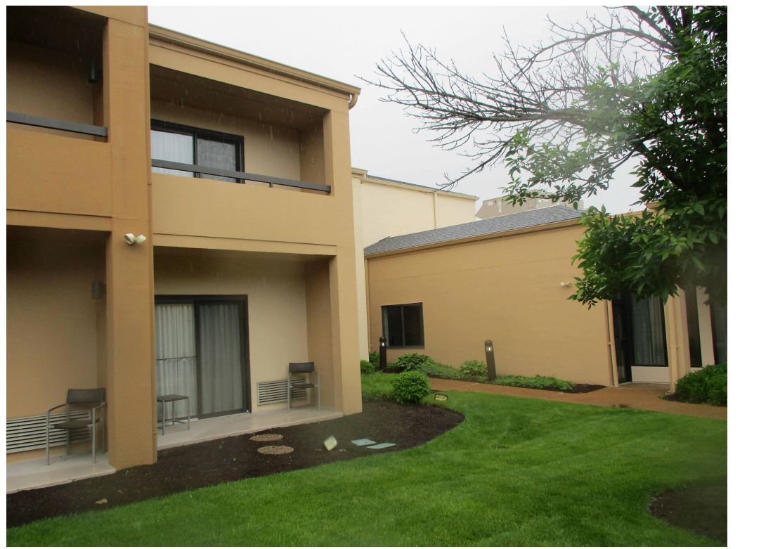
2 EXTERIOR PHOTOS - SOUTH COURTYARD 12" = 1'-0"
