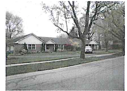
PHOTO OF EXISTING FRONT FACADE
